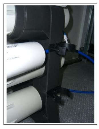
Attach the blue RO line from your Merlin-GP into one end of the UV filter. You will need to cut it to the length needed to make the bend into the UV filter. The other piece of blue tubing can be attached to the other end of the UV filter and will be your final product line.
