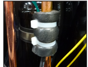
Figure 4: Thermistor attached to the refrigerant line.
