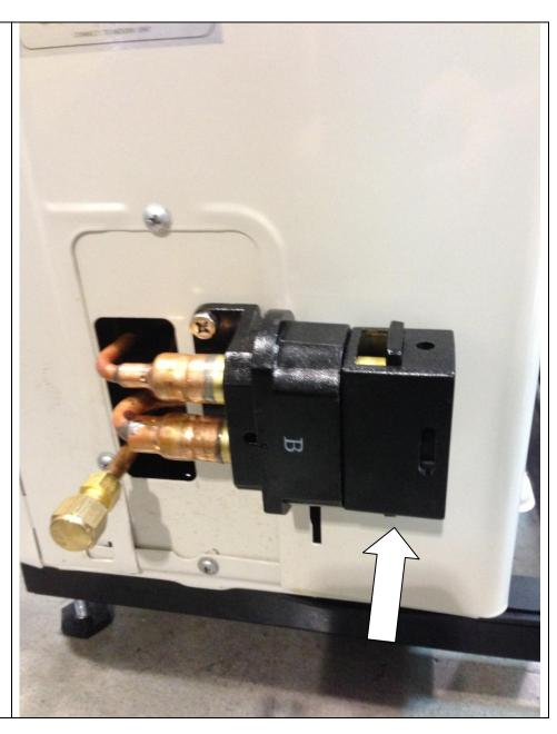
Pull back on release lever to release protective cap. Please keep clear of protective cap as it is under pressure and will release with some force.
