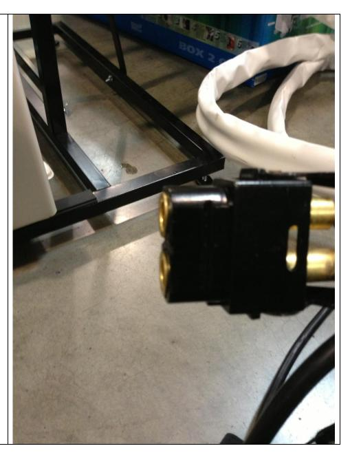
Insert indoor unit connector into the outdoor unit receptacle.
