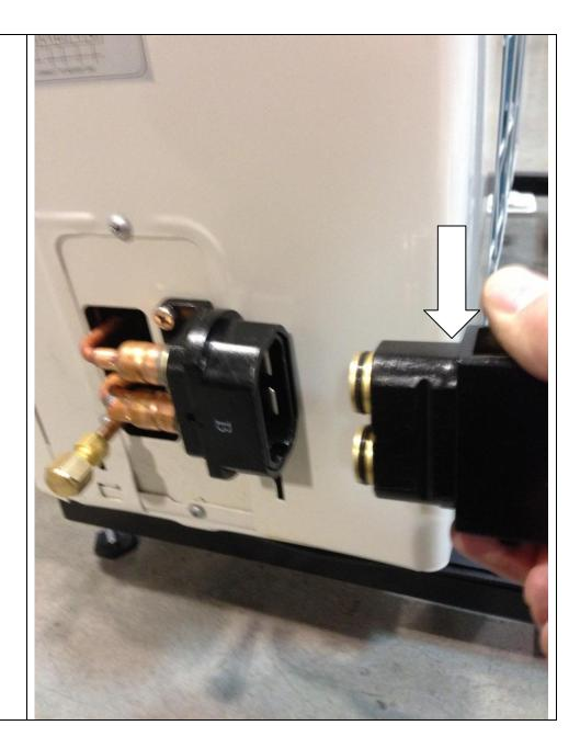
Remove dust cover from indoor unit connector.
